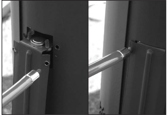
Figure 37: Spill switch installation.
