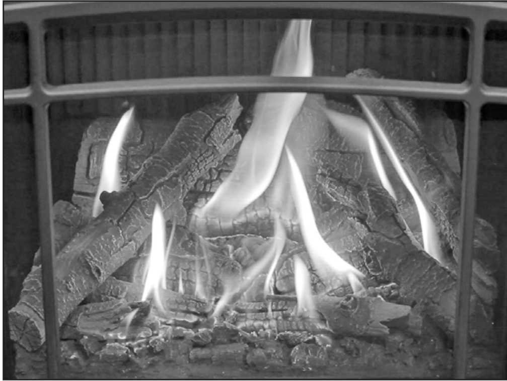
Figure 47. Proper Burn and Flame
