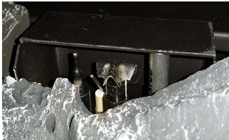
Figure 20: Pilot assembly beside the burner.
